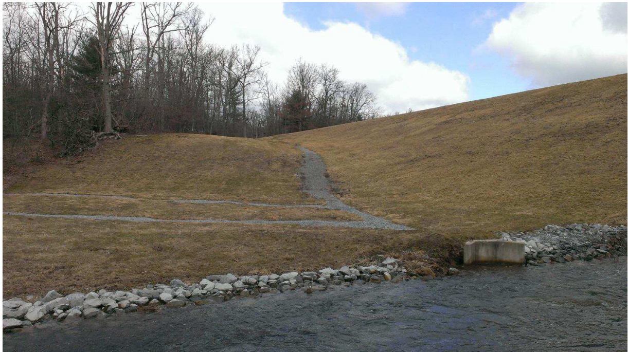
View of west side embankment
